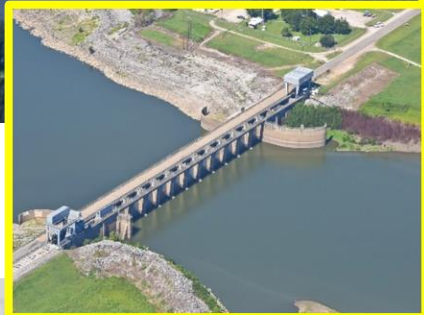
Low Sill Control Structure
