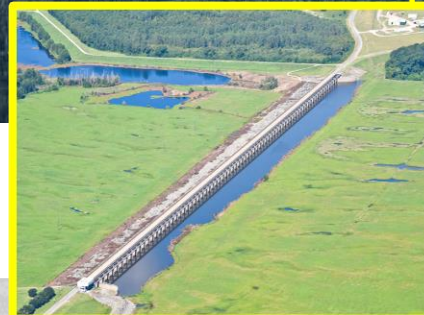
Overbank Control Structure
