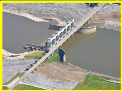
Auxiliary Control Structure
